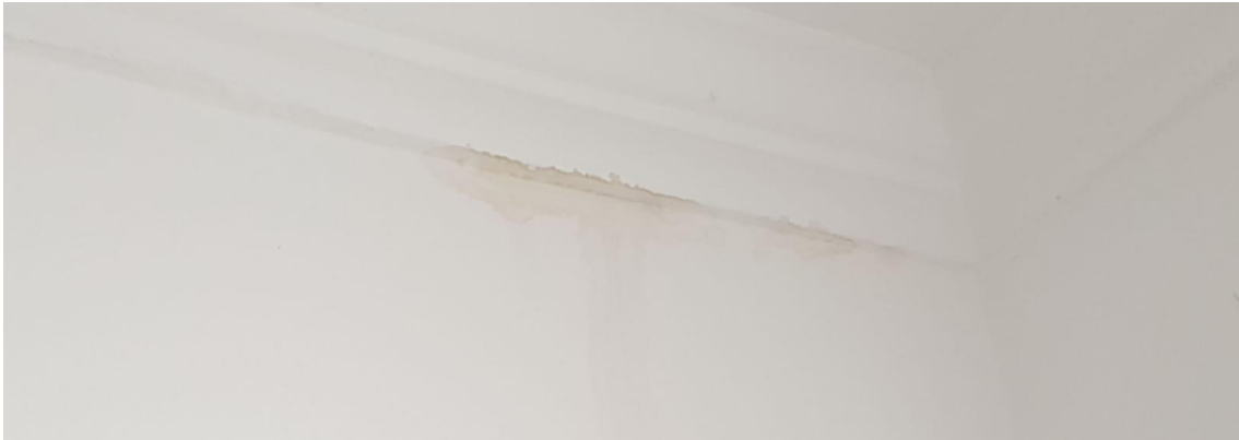
Figure 6 above: Water damage at 2F, 10 Randolph Crescent due to leaking roof.
