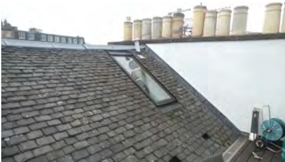
VIEW 20 Velux rooflight at roof terrace
